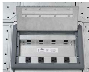
Recessed Data Center Floor Power Reception Point
